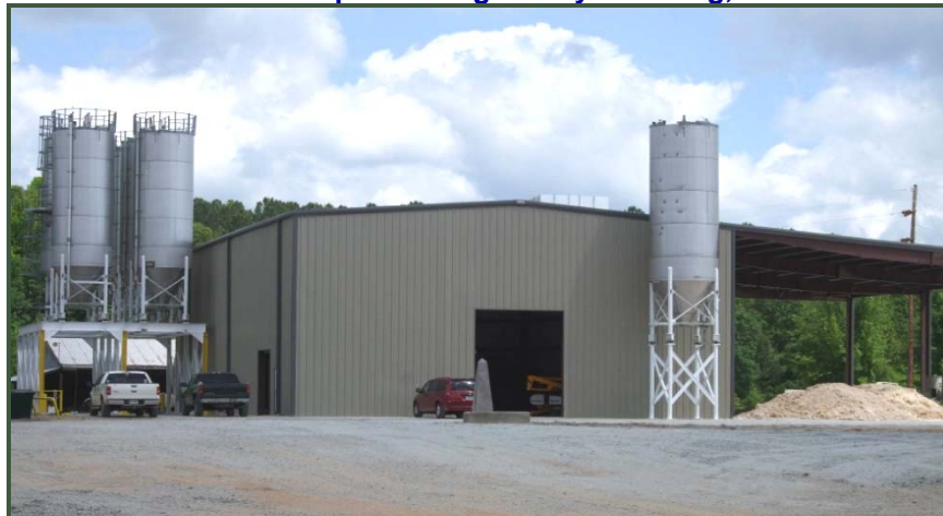
APM's new processing facility - Dearing, GA
